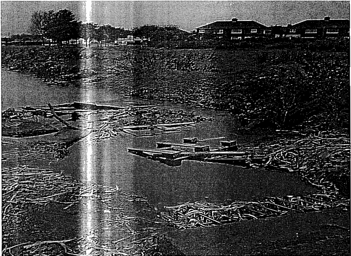
Surface Water Screen at Seagrang Park, Baldoyle.
