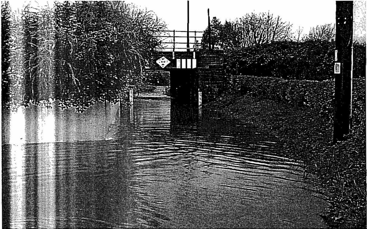
S.W. flooding at Railway in Ballisk.
