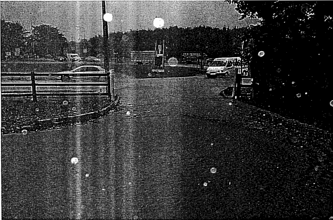
Flooding of Dublin/Belfast Roundabout at Little Chef
